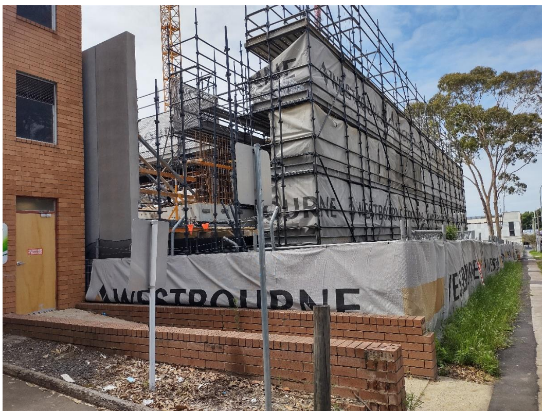
Photo 4: Construction south of site
